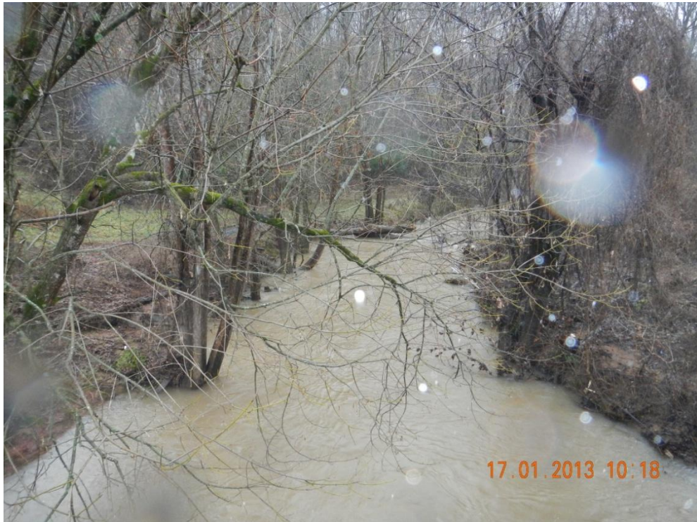
Photograph 3 – DSCN0021. N35.4325°, W-84.5859°. View of STR-1 (Oostanaula Creek) facing downstream and southwest at STA 95+81R.
